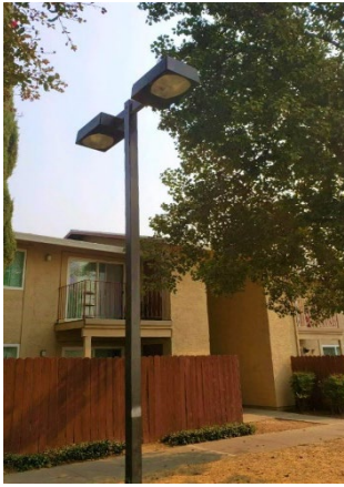
(2) LED Fixture Replacements
